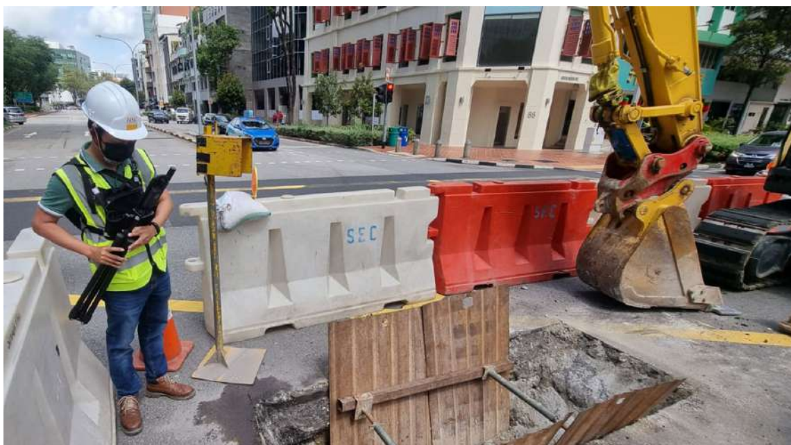
Figure 2: Laying pipelines - the viDoc helped collect data that was processed on PIX4Dcloud.
