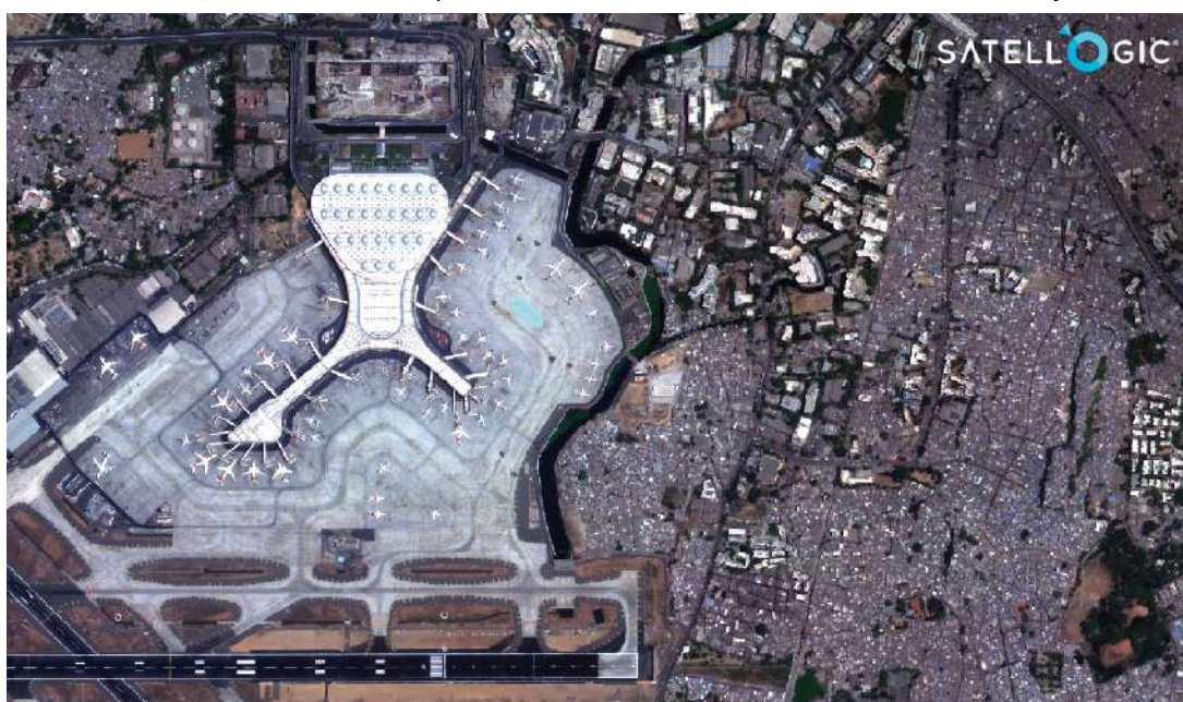
Figure 2: Mumbai Airport, India.
