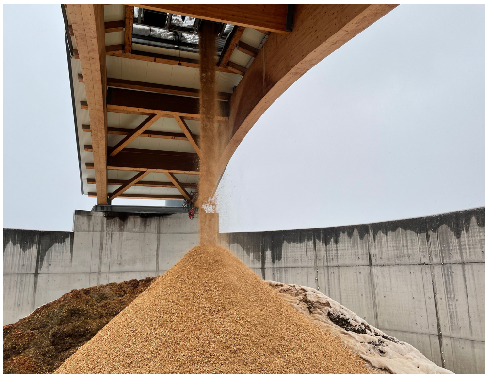
Figure 1: The BLK247 VolumeMonitor measures the volume of the grain silo even while the silo is being filled.
