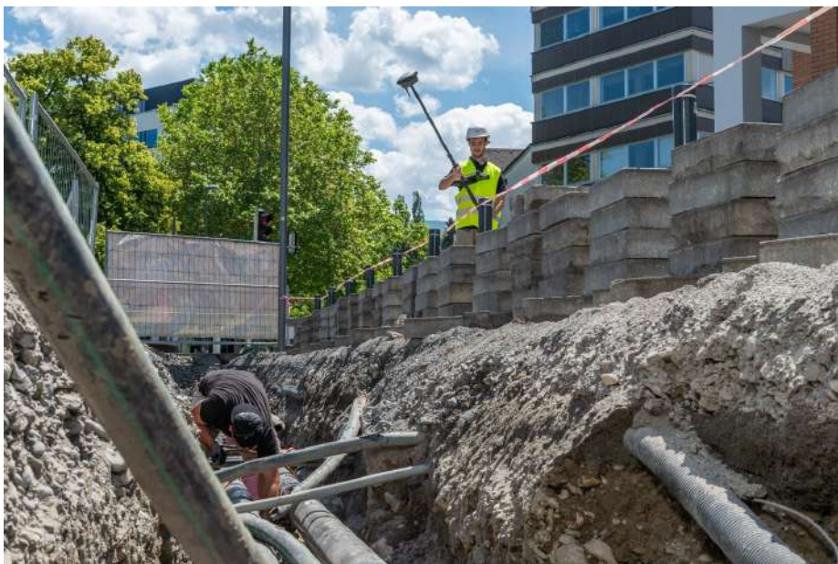
Figure 2: A versatile, survey-grade GNSS RTK rover with visual positioning helps surveying professionals to capture an environment in images quickly and decide which points to measure later.
